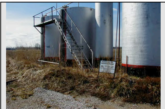
Typical tank battery
